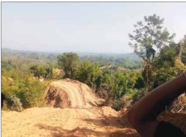
Photo: Ruilui-Bara Kamalak road in Sajek being constructed destroying gardens of indigenous villagers
